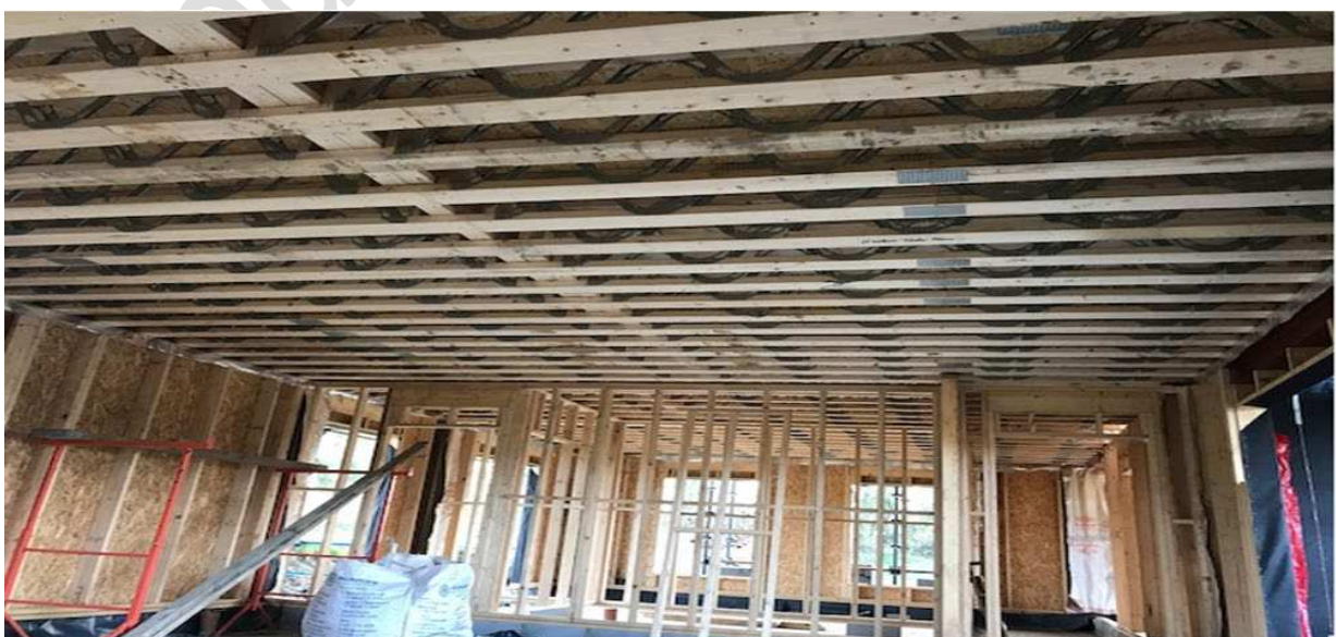
Modern Timber Frame
